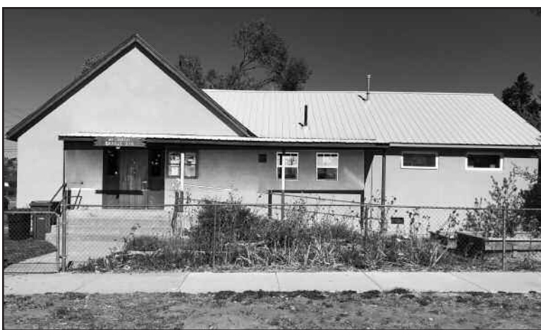
New windows and stucco on the building at Mount Lookout.
