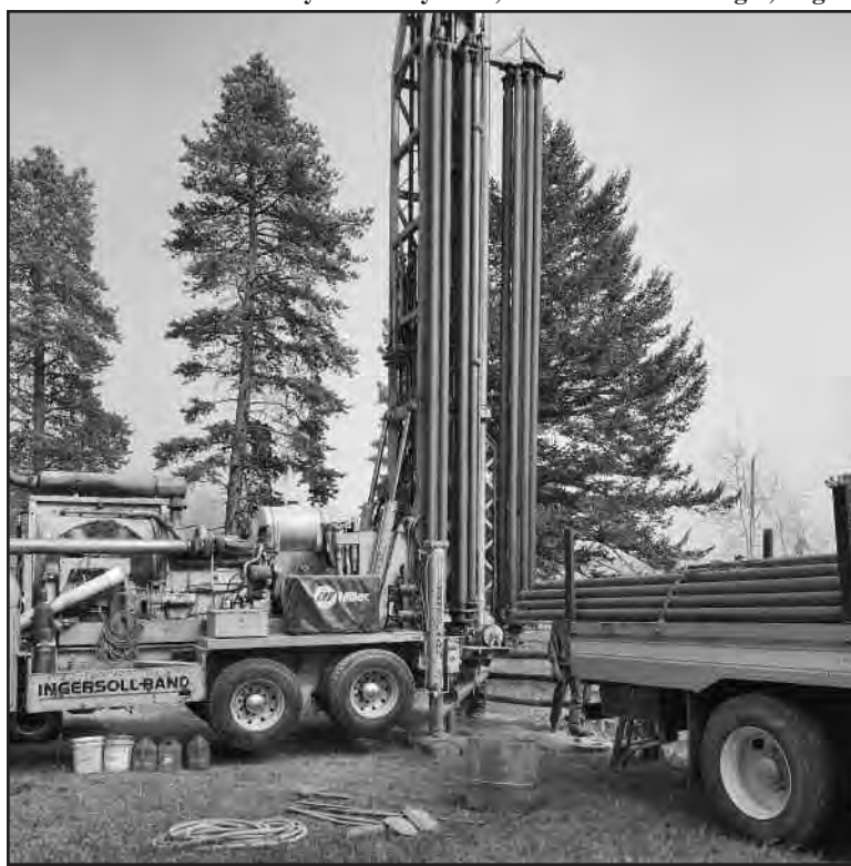
Drilling rig digging the new well for Pleasant Park Grange.
